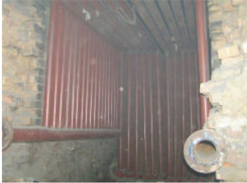
**Figure 1a: Installation of new bent-tubes**
